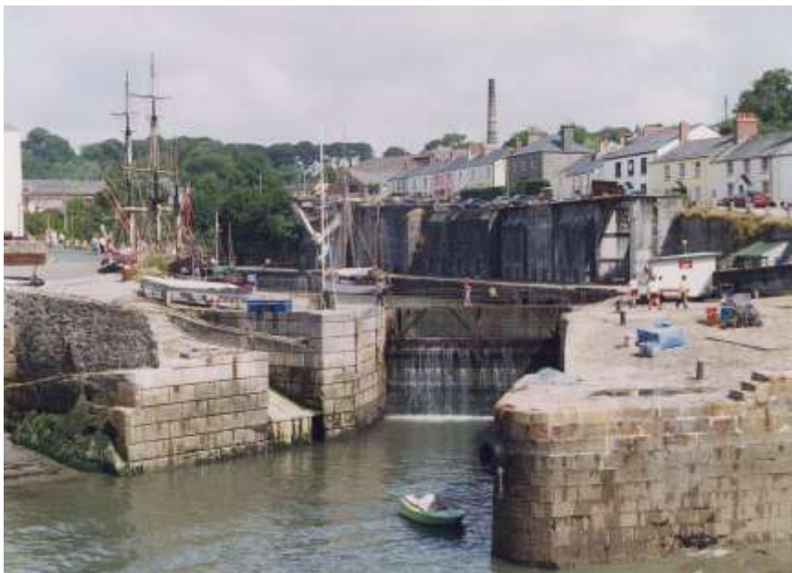
Charlestown Harbour. Storage bins for china clay on the right?
